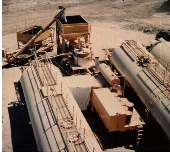
Figure 3-2 Asphalt Rubber Production Set Up at HMA Plant
