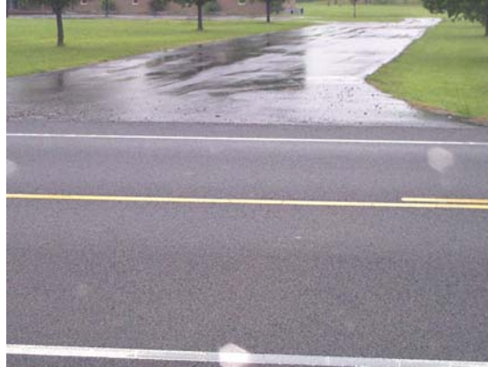
Figure 2-3 Free-Draining RAC-O Next To Dense-Graded HMA
