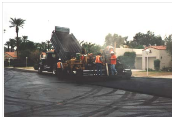
Figure 4-1 Unloading RAC-G into Paver Hopper
