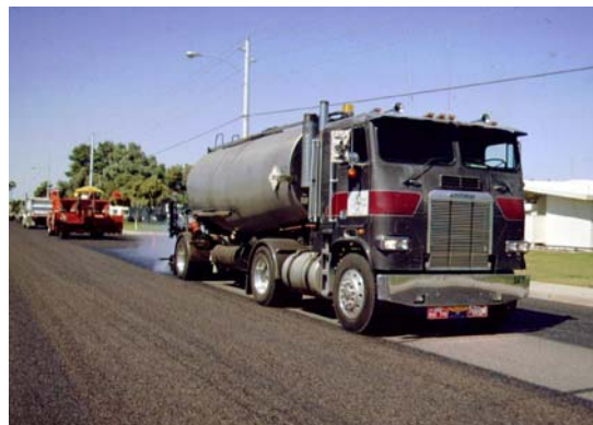
Figure 4-2 Chip Seal Train
