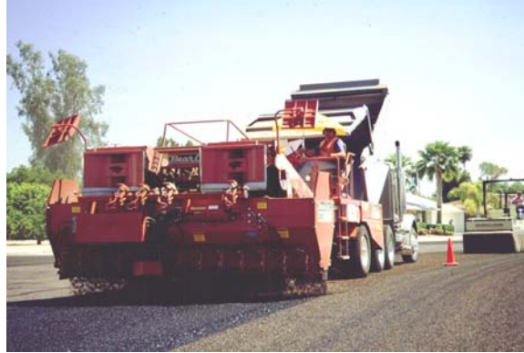
Figure 4-3 Spreading Precoated Aggregates
