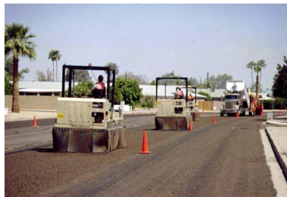
Figure 4-4 Rubber-Tired Rollers with Skirts on Chip Seal
