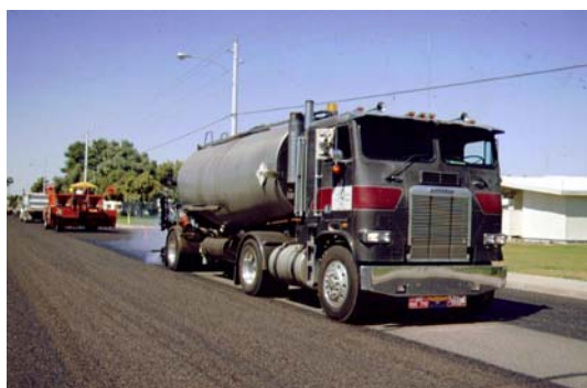
Figure 2-4 Chip Seal Train
