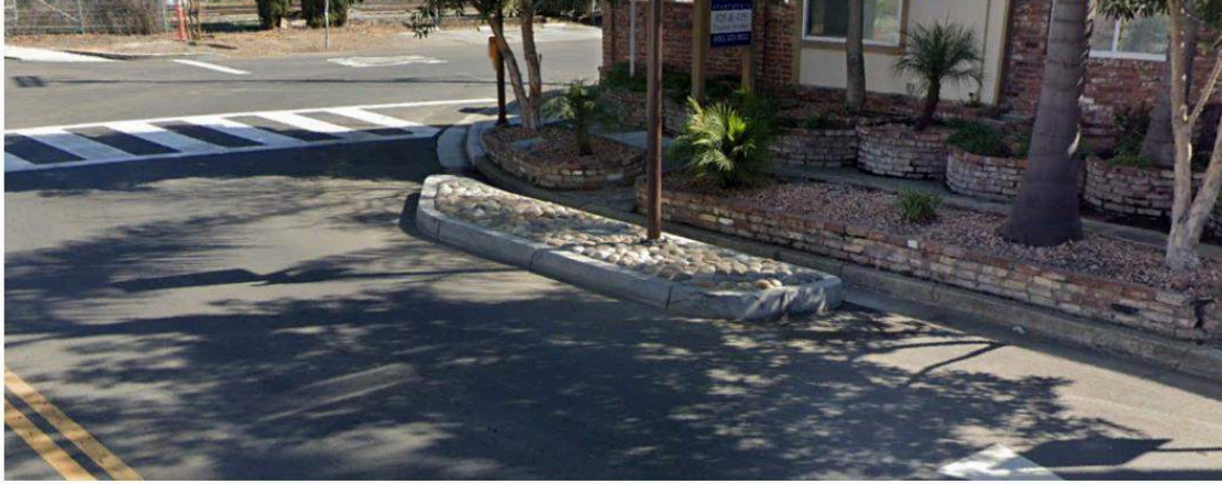
Example: Permanent tradition intersection bulbout (Location: Chilco St. at Hamilton Ave.)
