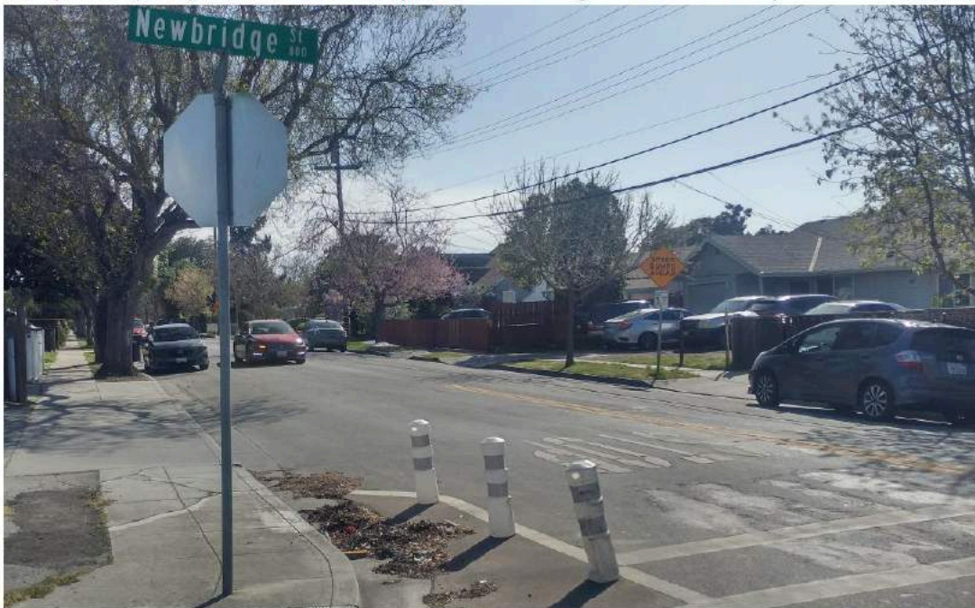
Example: Temporary intersection bulbout (Location: Newbridge St. at Carlton Ave.)
