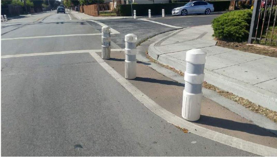
Example: Temporary intersection bulbout (Location: Newbridge St. at Carlton Ave.)
