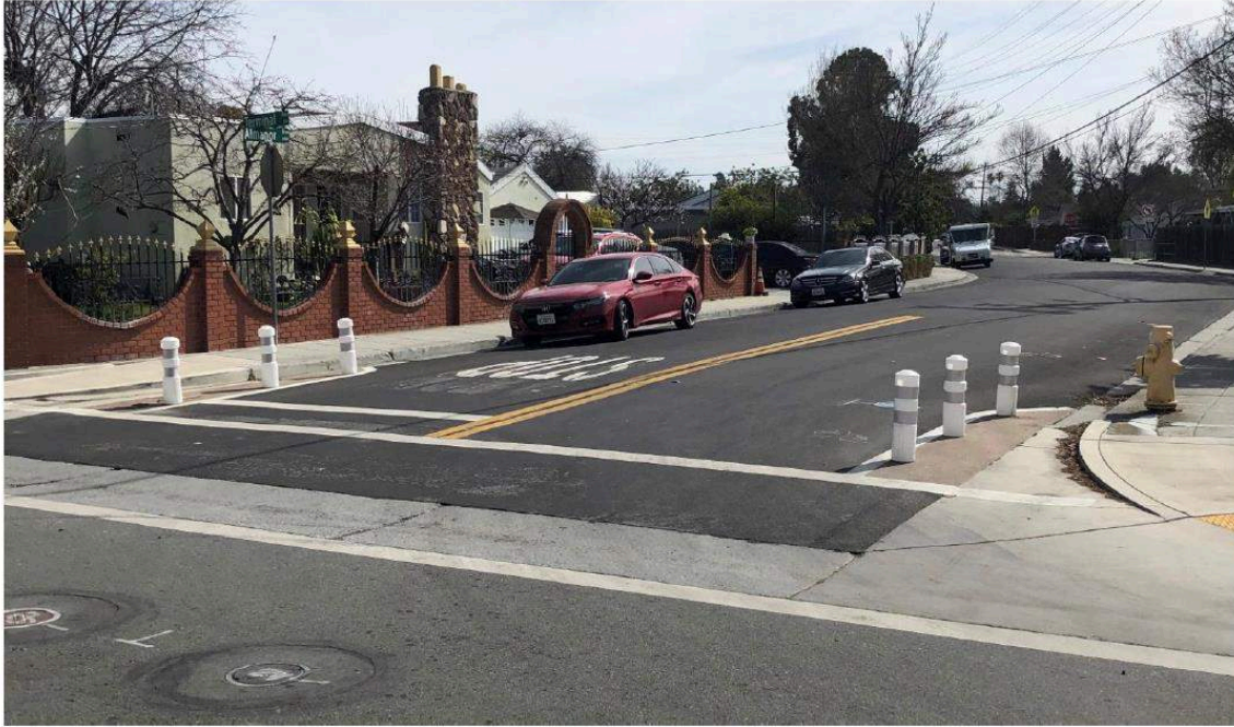
Example: Temporary intersection bulbout (Location: Almanor Ave. at Terminal Ave.)
