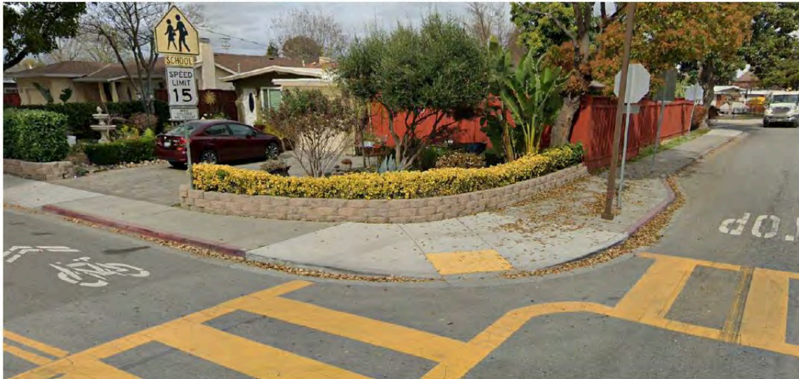
Example: Permanent tradition intersection bulbout (Location: Chilco St. at Hamilton Ave.)
