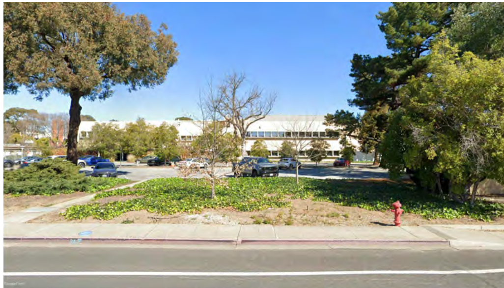
Figure 9: View on Laurel Street Toward East
