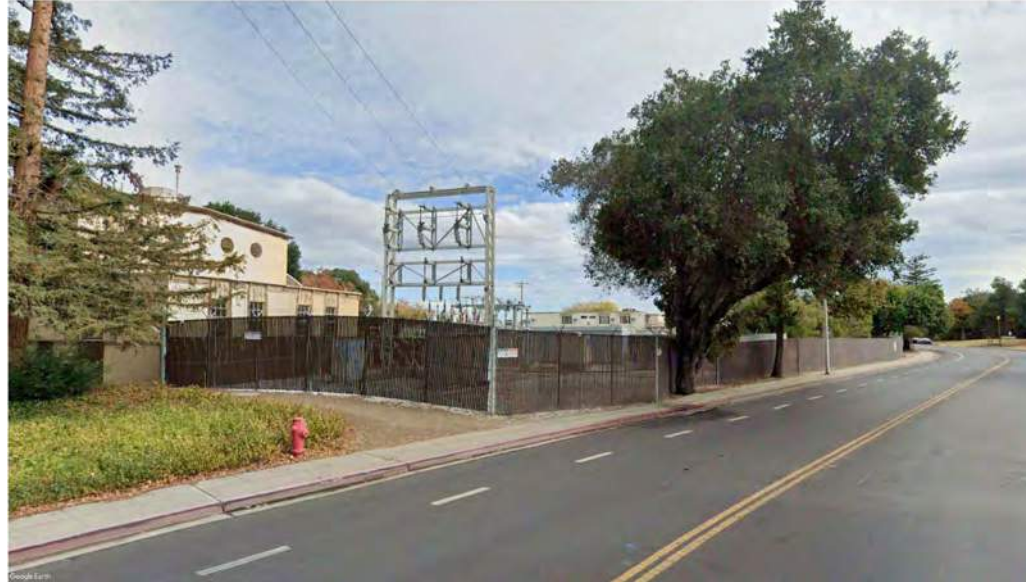
Figure 6: View on Laurel Street Toward South
