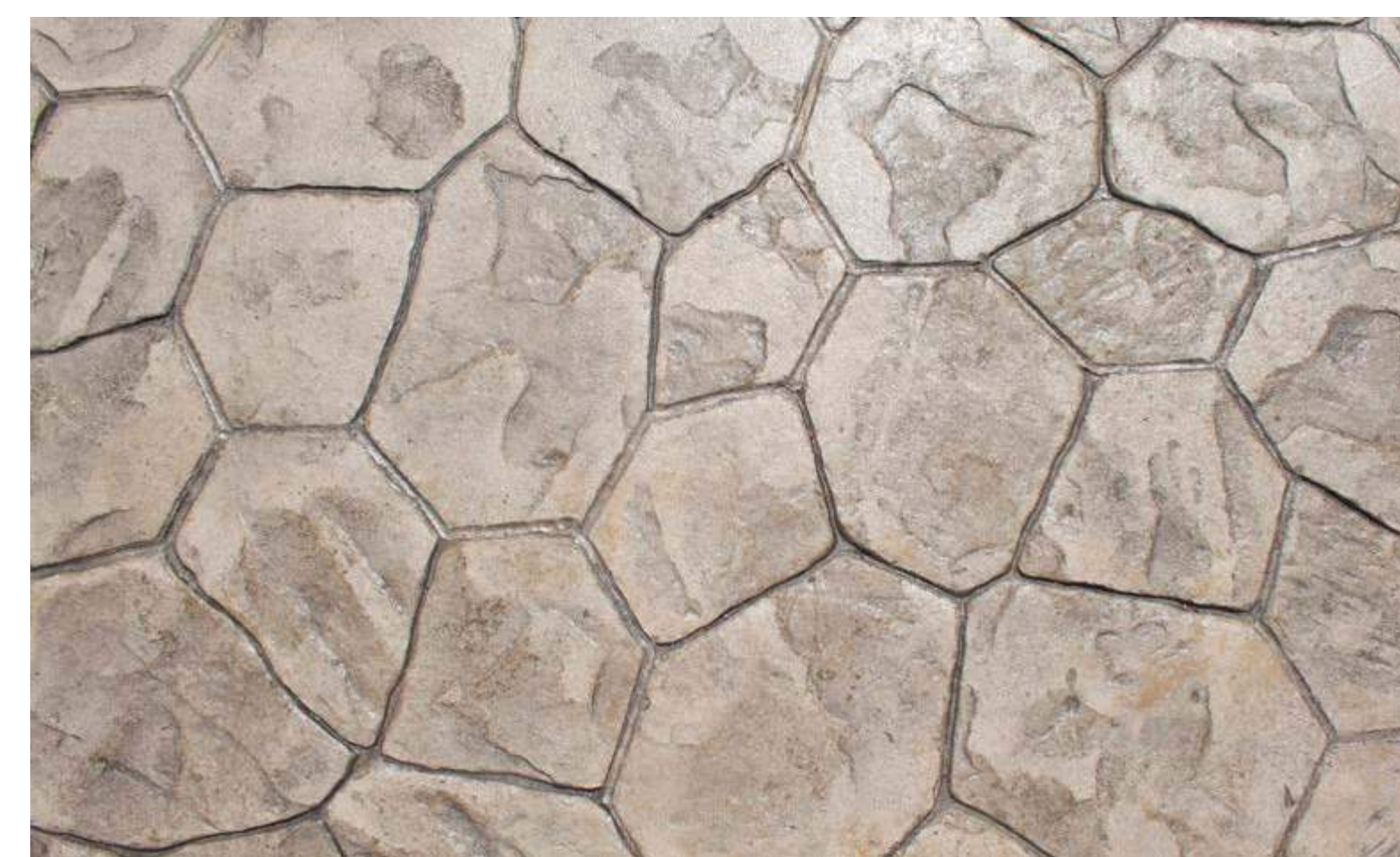
Pavement Node - Stamped Concrete
