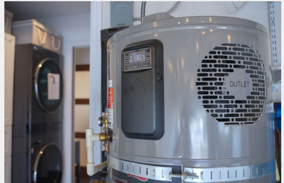
Heat pump water heater and electric dryer
