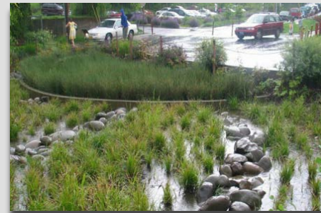
Example 3: Bioretention Area
