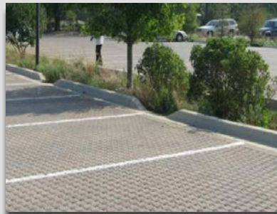
Example 2: Permeable paver w/ swale
