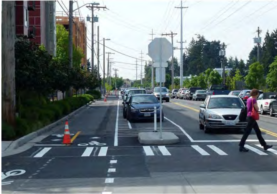
Figure 5-17 Existing one-way bike lane
