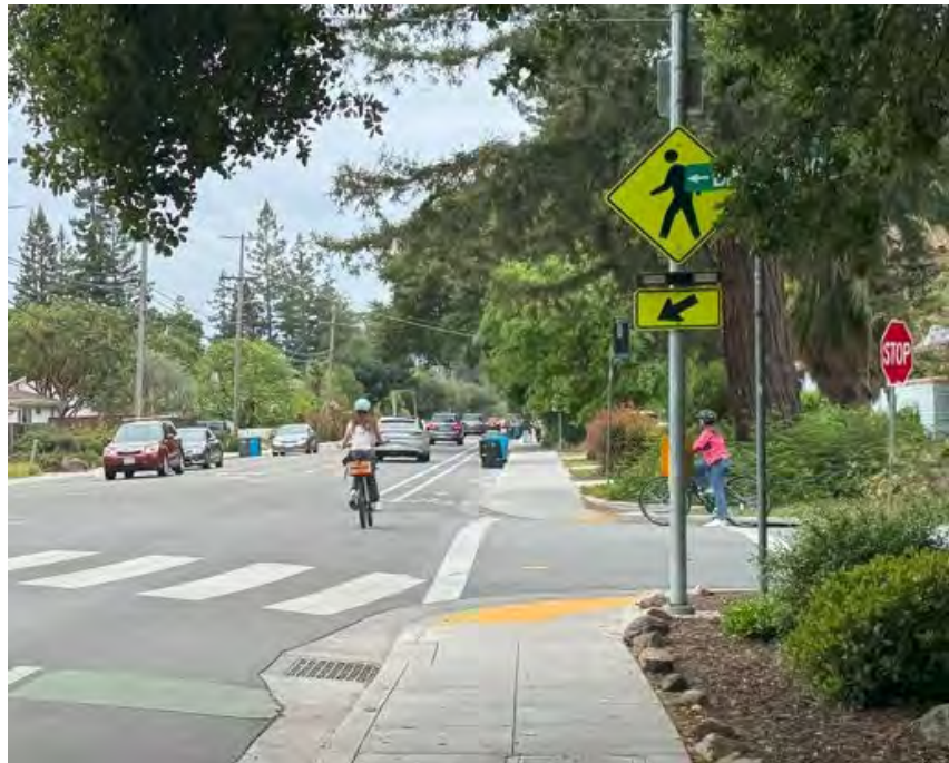
Figure 5-16 Trees blocking street sign
