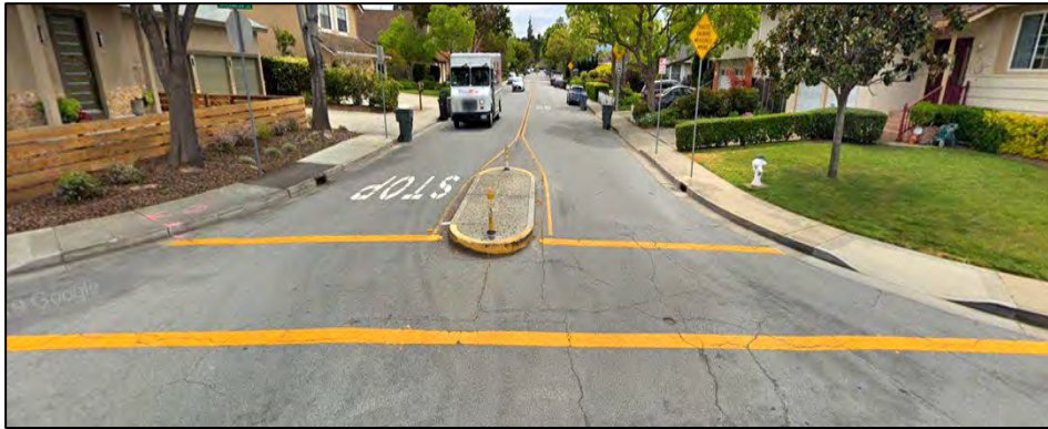
Figure 5-5 Median Island on residential street
