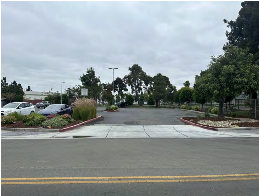
Existing condition at 4085 Campbell Avenue (facing Scott Drive) - Northern driveway
