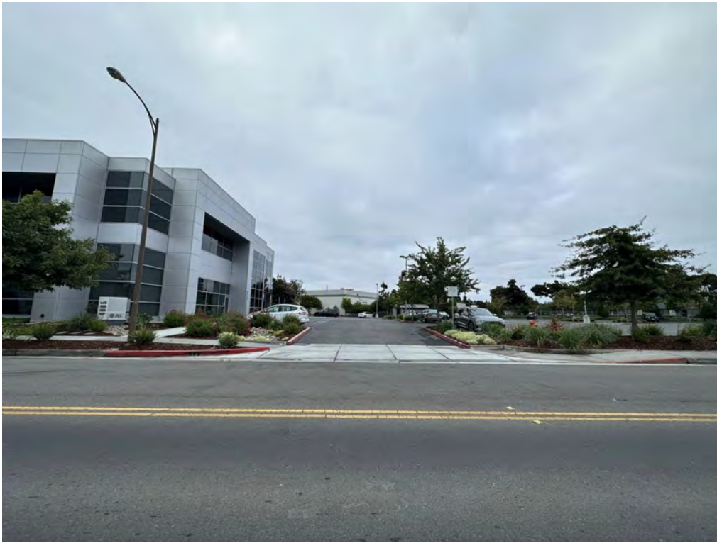
Existing condition at 4085 Campbell Avenue (facing Scott Drive) - Southern driveway
