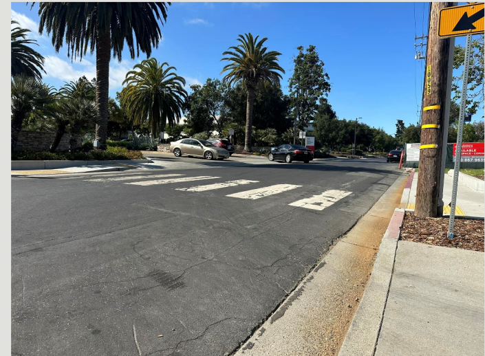
Right of driveway (~ 50' of existing red curb)
