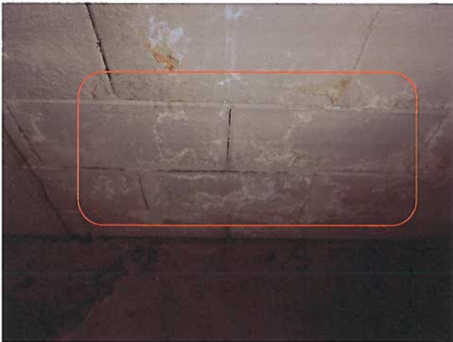
Figure 3 Efflorescence bloom on the CMU foundation wall along El Camino Real.
