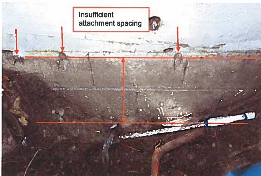
Figure 23 DT location at the CMU foundation wall at the rear of the garage. Note that the wall waterproofing has slipped down - leaving a portion of the wall unprotected. Additionally, note the insufficient attachment spacing.
