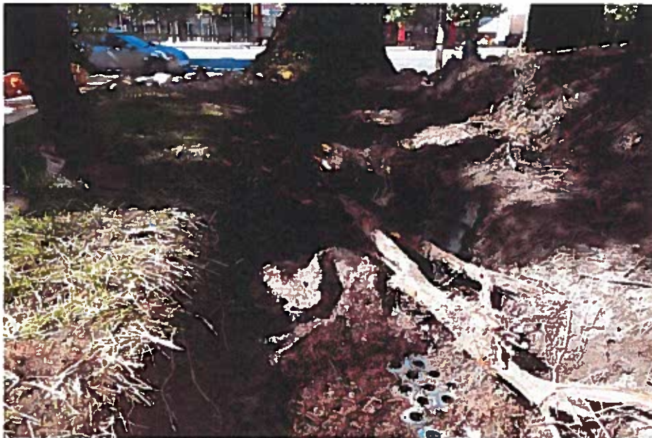
Figure 10 DT location showing large root system extending throughout the podium area. Root system is damaging the waterproofing membrane through surface abrasion and by penetrating the membrane - opening pathways for water intrusion into the podium slab.
