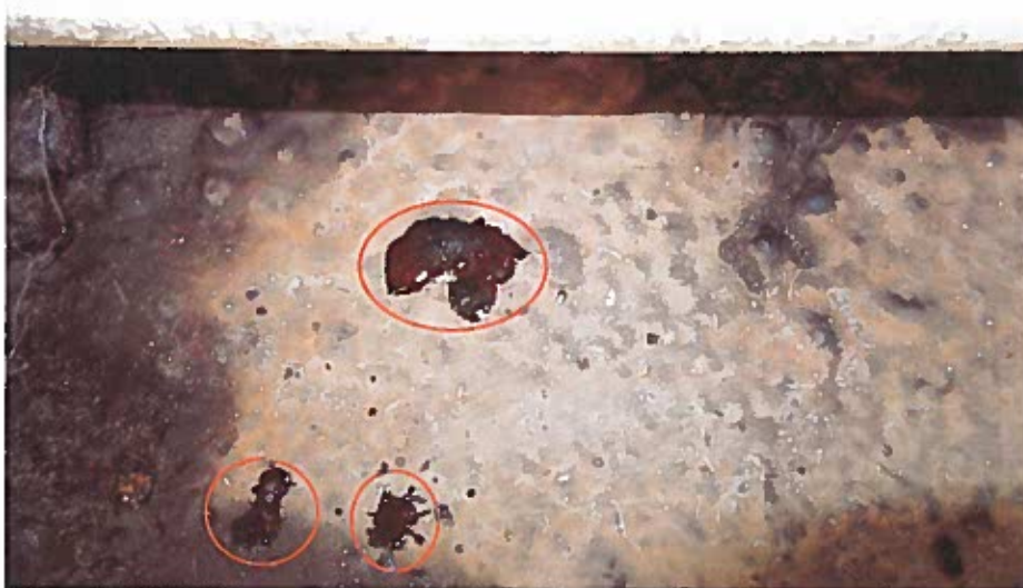
Figure 16 Sliced blisters seeping trapped water that was below the waterproofing – indicating that moisture is moving through the waterproofing membrane.
