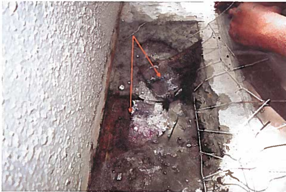
Figure 22 Note moisture below membrane, indicating water intrusion is occurring. Water below the waterproofing membrane can travel through voids and unadhered portions of the membrane.
