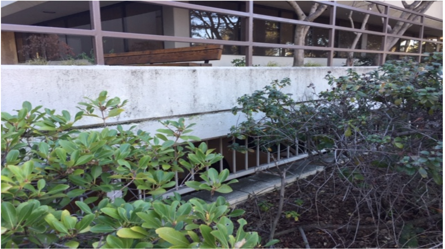
North Edge of the Podium partially supporting the West Building The open grille with vertical bars ventilates the parking space below the Podium.
