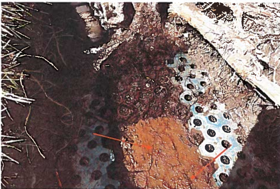
Figure 9 Destructive testing (DT) area where grass, soil, etc. to expose waterproofing. Note how the small root hairs are embedded within the waterproofing membrane.
