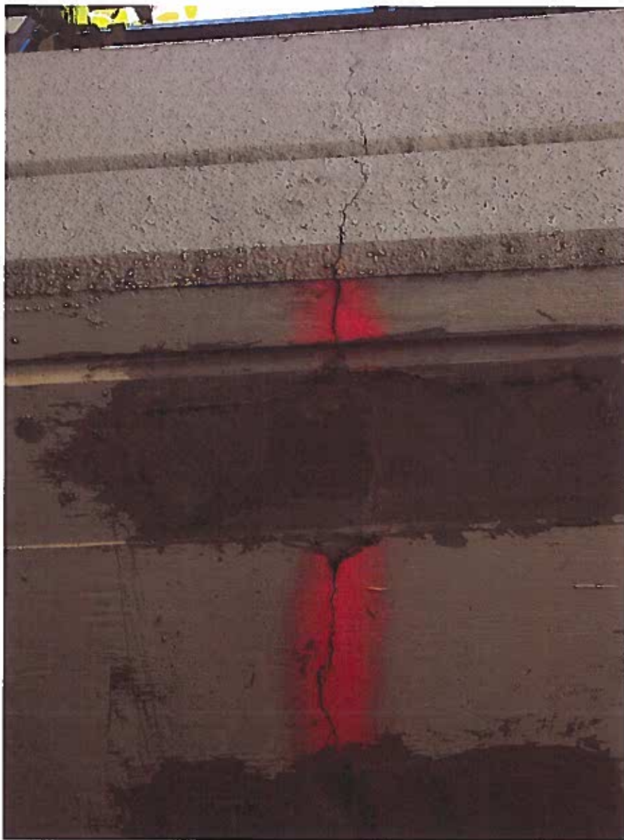
Photo 1 – Podium slab cracks along with chip and patch regions at gridlines 2.5/H1
