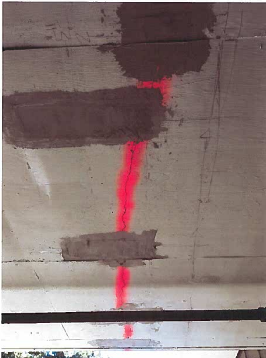
Photo 3 - Podium slab cracks along with chip and patch regions at gridline 2.5
