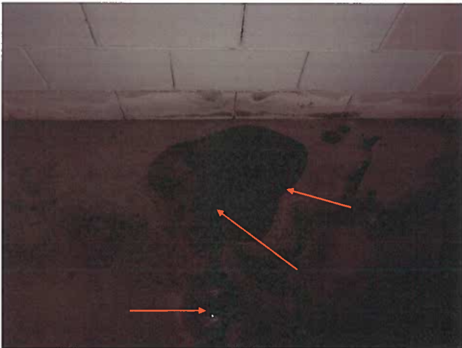
Figure 5 Water with rust staining from podium slab leak above.
