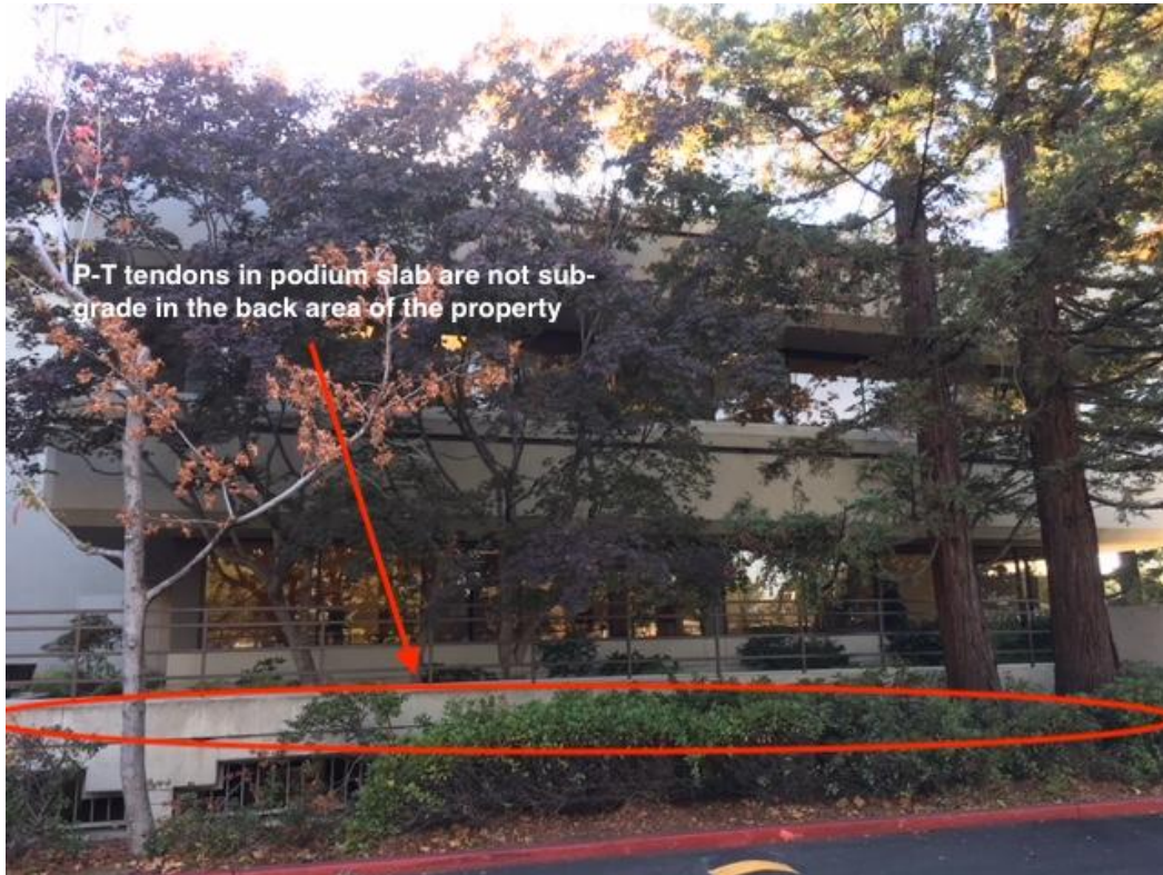
A-1.9 – View on the north side of the 1000 El Camino Real building showing that the Post tension (P-T) tendons are above grade, which is a different condition than in the front.
