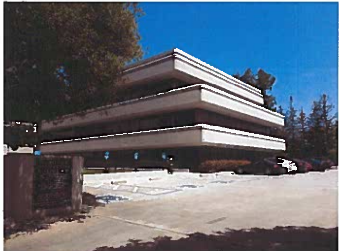
Figure 1 Menlo Park Office Center
