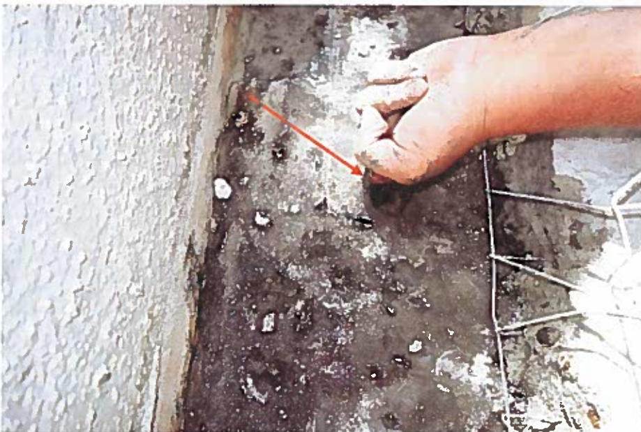
Figure 21 Note the void in the membrane where it is unadhered to the slab below.
