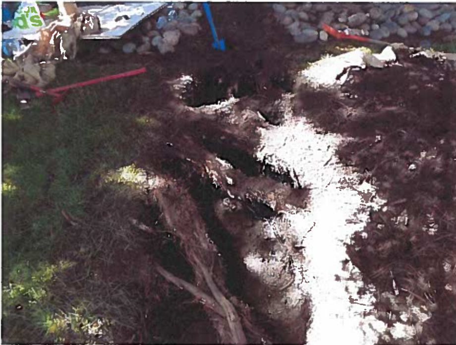
Figure 12 Large roots extending from trees along El Camino Real toward the building (above the podium area.) These roots are throughout the podium.
