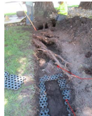
THICK TANGLE OF TREE ROOTS OVER THE PODIUM AND UNDERGROUND GARAGE
