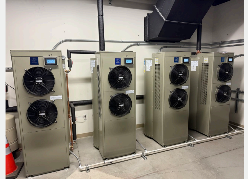
Completed installation of heat pump water heaters for Burgess Pool showers
