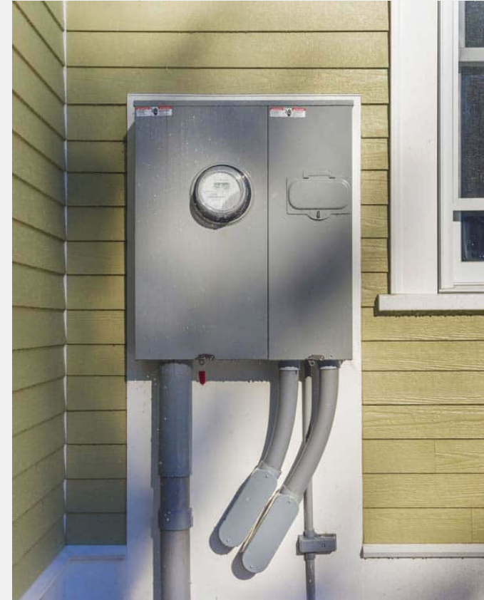
Residential electrical panel and meter
