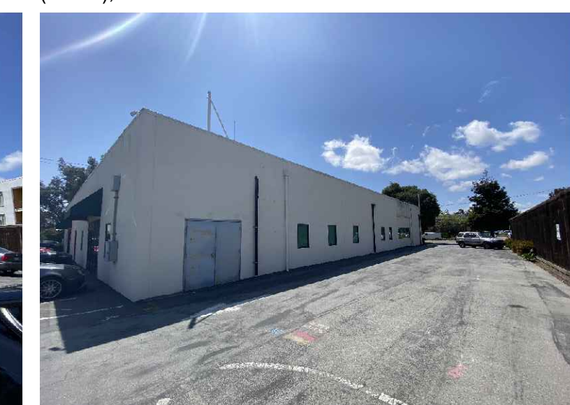
8. VIEW FROM NW PORTION LOOKING SW
