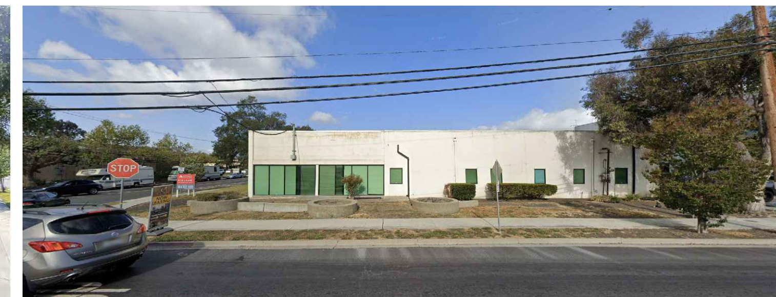
4. VIEW FROM HAVEN AVENUE (EAST)
