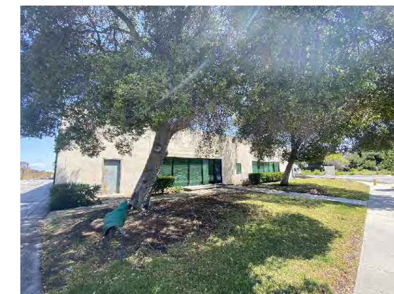
3. VIEW FROM HAVEN AVENUE (SOUTH), SW CORNER OF SITE
