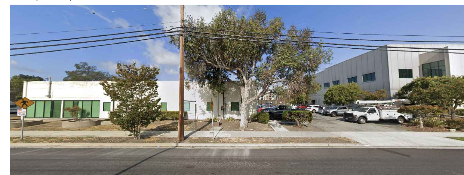
5. VIEW FROM HAVEN AVENUE (EAST)
