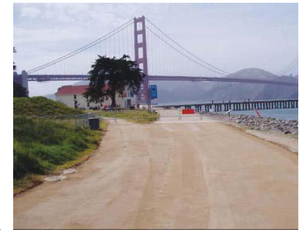
Natural-Looking Treated Trail Pavement
