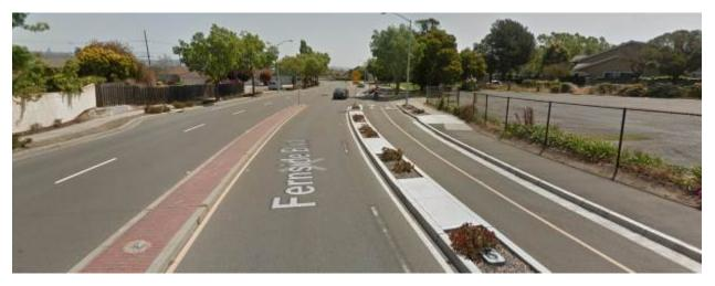
Figure 12 Two Way Cycle Track (Fernside Boulevard, Alameda)
