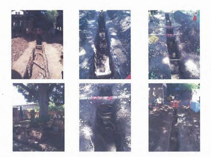
As you can see from the images there are some 2" diameter roots in the areas where the proposed foundations would go. We have spoken with the Project Engineers and are assured that the vast majority of these roots can be retained with the use of a pier and grade beam foundation system.
