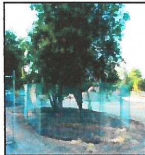
IMAGE 2.15-1 Tree Protection Fence at the Dripline
