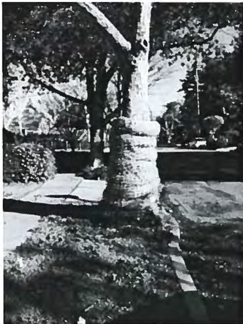
Example of straw wattle and orange plastic type protection.
