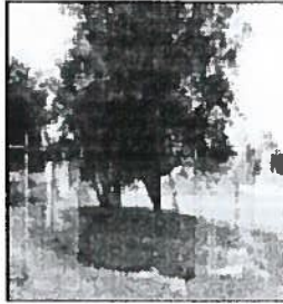
IMAGE 2.15-1 Tree Protection Fence at the Dripline
