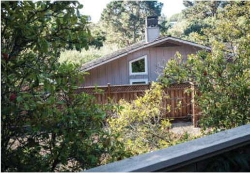
NEIGHBOR'S HOME - SIMILAR WINDOW ADDED TO LIVING ROOM
