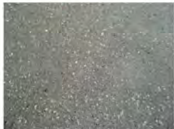
HEAVY SANDBLAST CONCRETE PAVING
