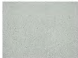
LIGHT SANDBLAST CONCRETE PAVING
