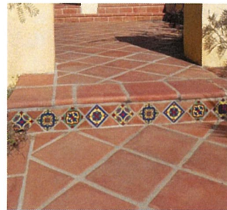
TERRACE PAVING, TYP. (BLDG. 1, 2 & 3) SALTILLO TILE
