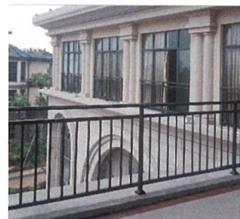
WROUGHT IRON RAILING (BLDG. 1, 2 & 3)
