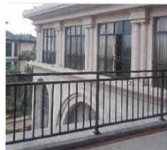
WROUGHT IRON RAILING (BLDG. 1,2 & 3)
