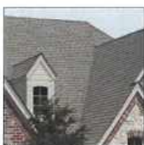
8 COOL WEATHERED ROOF
