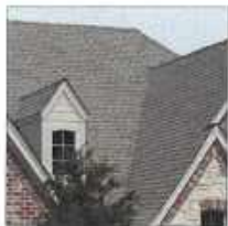
9] COOL WEATHERED ROOF
