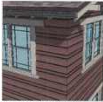
4] CEMENTITIOUS HORIZONTAL SIDING
