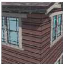
4 CEMENTITIOUS HORIZONTAL SIDING
