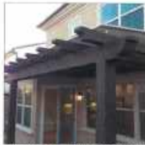
8] TRELLIS (ENTRY WAY AND COMMON AREAS)
