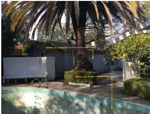
6 EXISTING SOUTH EAST FACE OF GARAGE
