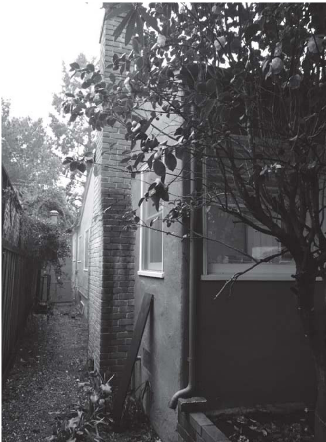
SIDE YARD VIEW OF EXISTING HOUSE - NORTH 2 SITE PHOTO NOT TO SCALE
