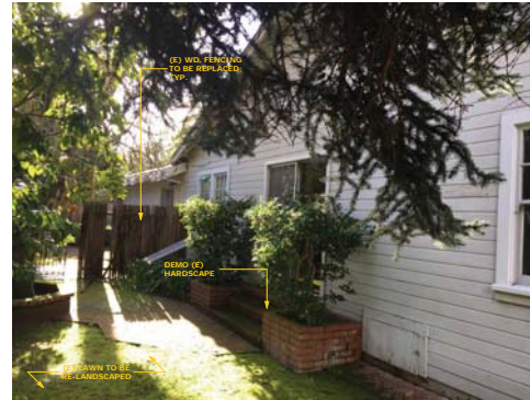
5 EXISTING NORTH EAST FACADE
