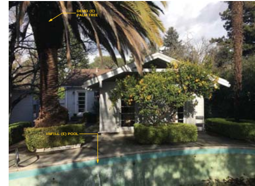
3 EXISTING SOUTH FACADE
