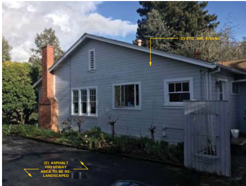
7 EXISTING WEST FACADE
