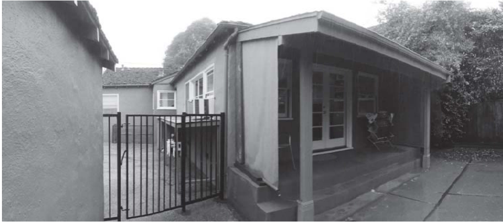
BACK YARD VIEW OF EXISTING HOUSE - SOUTH
