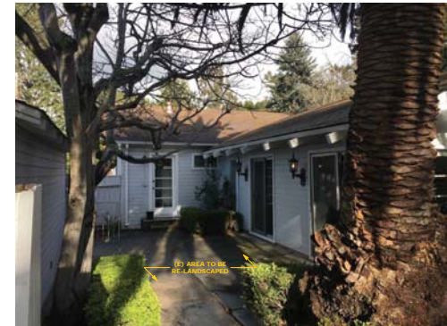
2 EXISTING SOUTHWEST FACE
