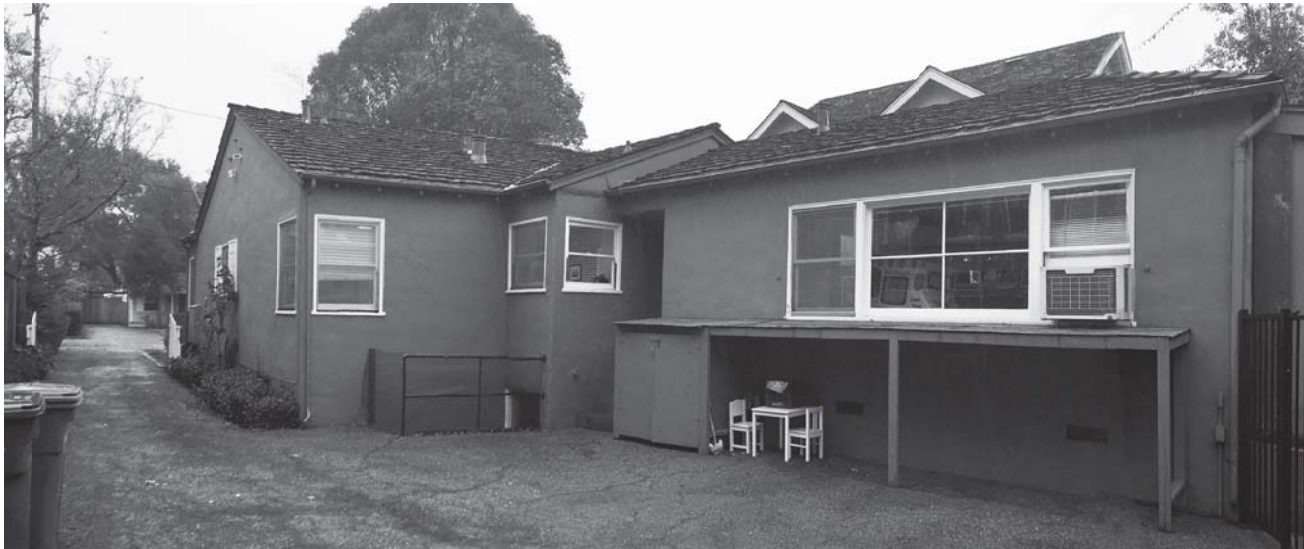
SIDE YARD VIEW OF EXISTING HOUSE - SOUTH
