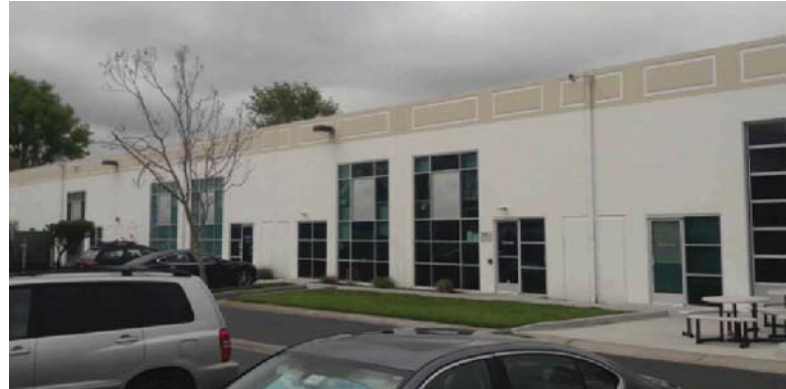
EAST SIDE OF BUILDING
