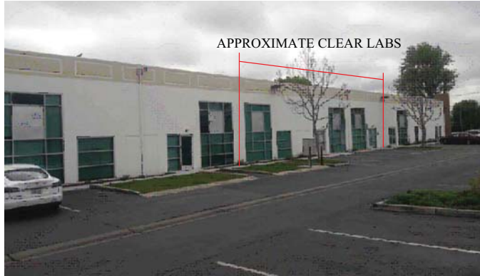
WEST SIDE OF BUILDING
