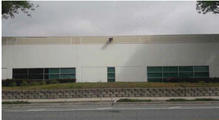
SOUTH SIDE OF BUILDING
