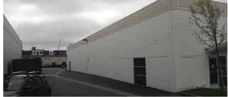
NORTH SIDE OF BUILDING
