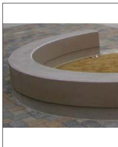
SEATWALL MADE ON SITE, WATER WASHED FINISHED
