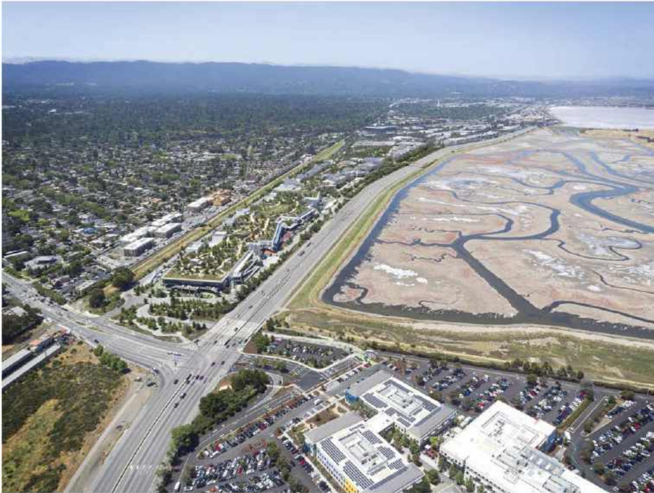
FACEBOOK CAMPUS AERIAL VIEW FROM EAST
