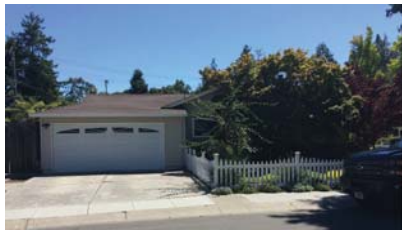
EXISTING 1008 GREENWOOD DRIVE (HEDGE RD. ELEVATION)
