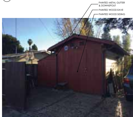
① EXISTING GARAGE ELEVATIONS - HAIGHT ST. 1:137.14
