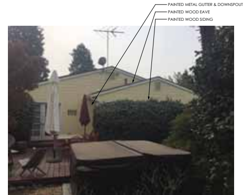
③ EXISTING MAIN RESIDENCE ELEVATIONS - REAR 1:137.14
