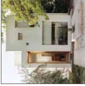
3 SMOOTH FINISH STUCCO: STEEL TROWEL SMOOTH COLOR INTEGRATED STUCCO COLOR : BENJAMIN MOORE - TBD
