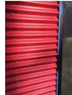
CORRUGATED SIDING - COLOR 1.8.D. ORIENTED VERTICALLY FOR ELEVATIONS W/ FASTENERS AS SHOWN ABOVE @ 24" OC.
