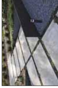
1 CONCRETE PAVERS: VARIOUS SIZED ARCHITECTURAL GRADE SMOOTH CONCRETE PAVERS WITH LIGHT FINISH
