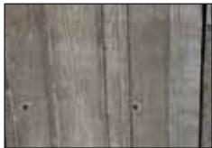
BOARD FORM CONCRETE: [ 8 ] 2" x 8" WOOD GRAIN, ARCHITECTURAL GRADE
