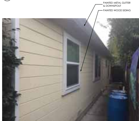
④ EXISTING MAIN RESIDENCE ELEVATIONS - WEST SIDE 1:137.14
