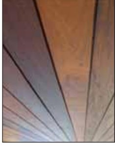
4 SHIPLAP WOOD SIDING: 1 x 6 CEDAR WOOD SIDING COLOR: SEMITRANSSPARENT SATIN
