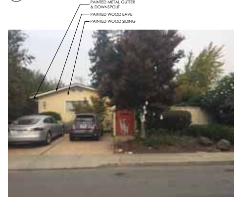
① EXISTING MAIN RESIDENCE ELEVATIONS - CHESTER ST. 1:137.14
