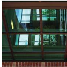
ALUMINUM STOREFRONT WITH CLEAR GLAZING MANUFACTURER: KAWNEER MANUFACTURER COLOR: BROWN MATERIAL: ALUMINUM ARCHITECTURAL FINISHES FRAME COLOR: BROWN
