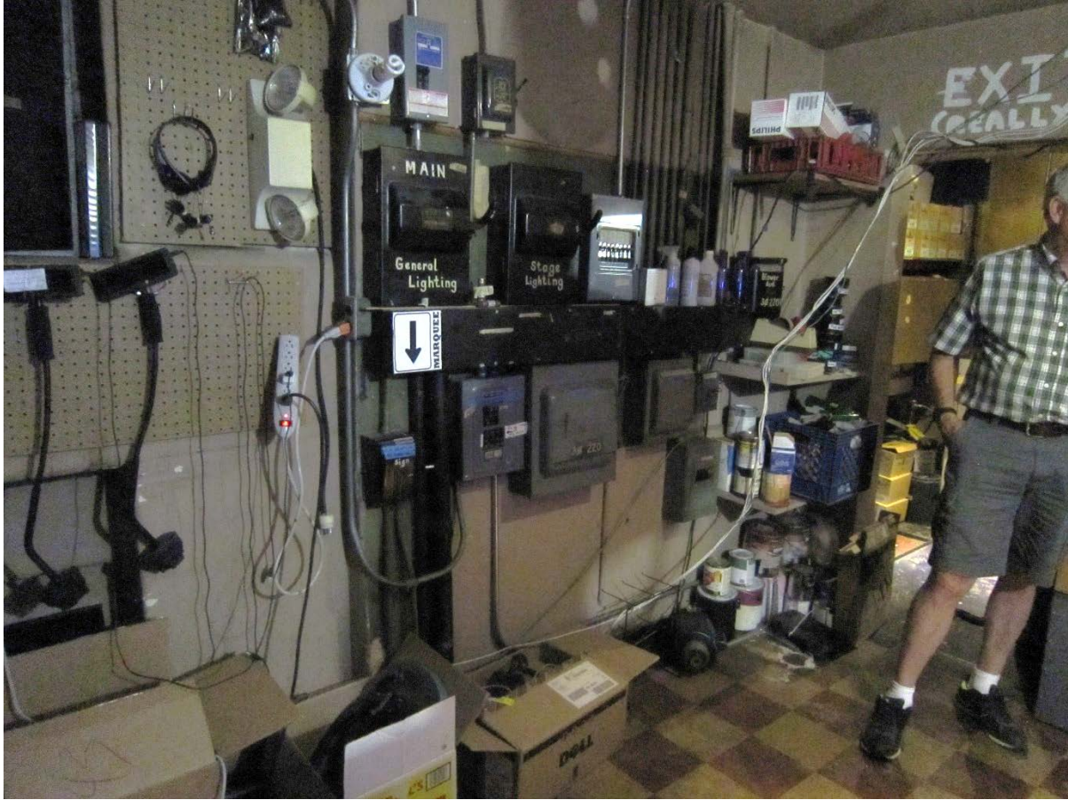
Photograph 8 – 949 El Camino Real- The Guild Theater
