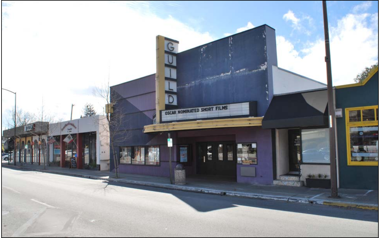
Figure 4: View southeast towards theatre
