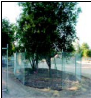
IMAGE 2.15-1 Tree Protection Fence at the Dripline
