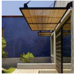
PHENOLIC WOOD AND METAL AWNING 8
