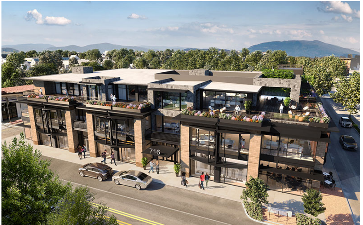
below: "Village on the roof" enriches the fabric of the city (please see sightline studies included in the planning set showing no visual impact from rooftop mechanical equipment & skylights).
