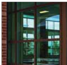
ALUMINUM STOREFRONT WITH CLEAR GLAZING
