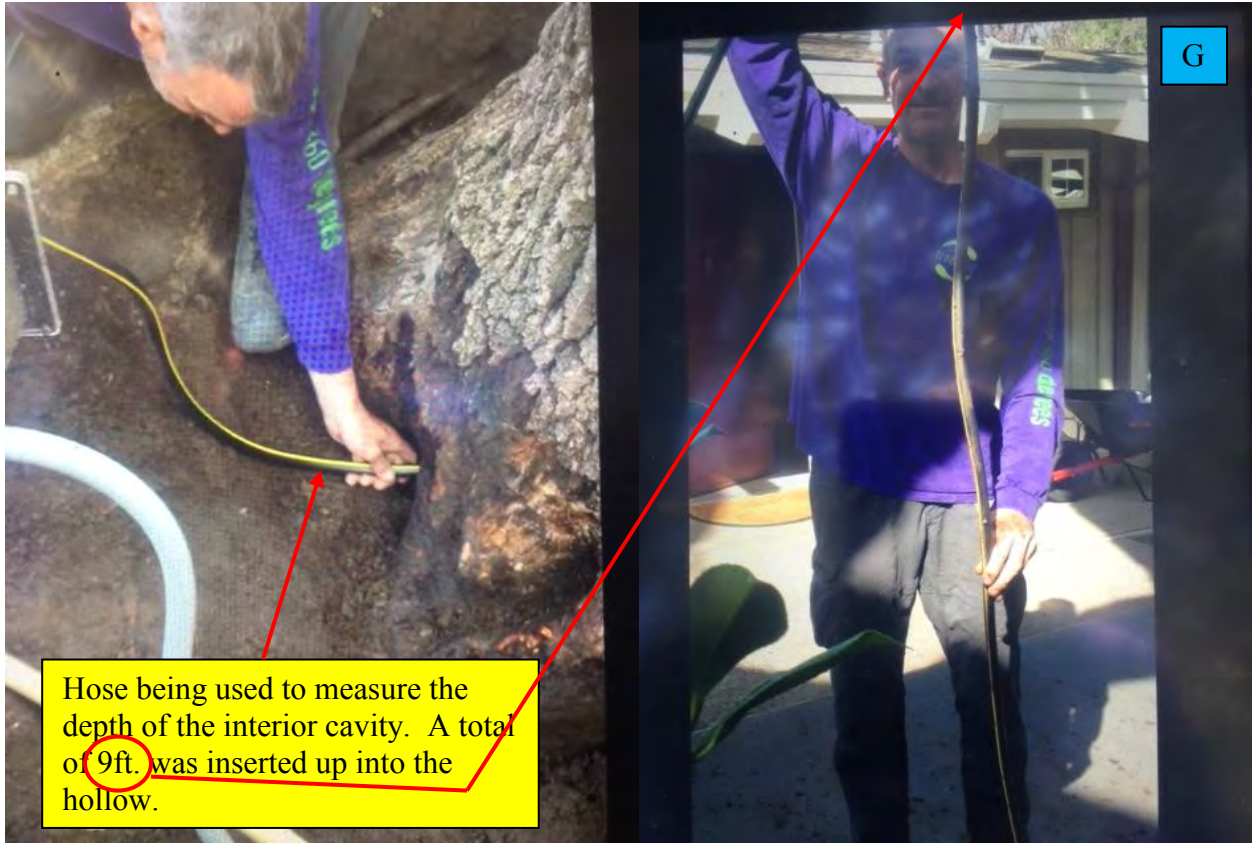
Photo G Hose used to measure depth of cavity.
