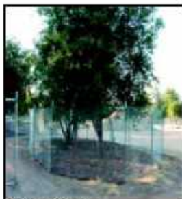
IMAGE 2.15-1 Tree Protection Fence at the Dripline
