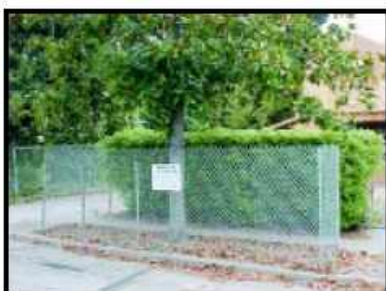
IMAGE 2.15-3 Tree Protection within a Planter Strip
