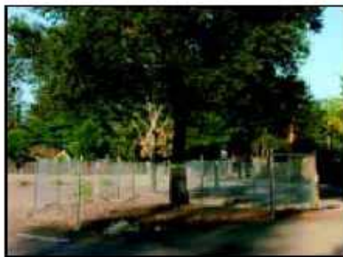
IMAGE 2.15-2 Tree Protection Fence at the Dripline
