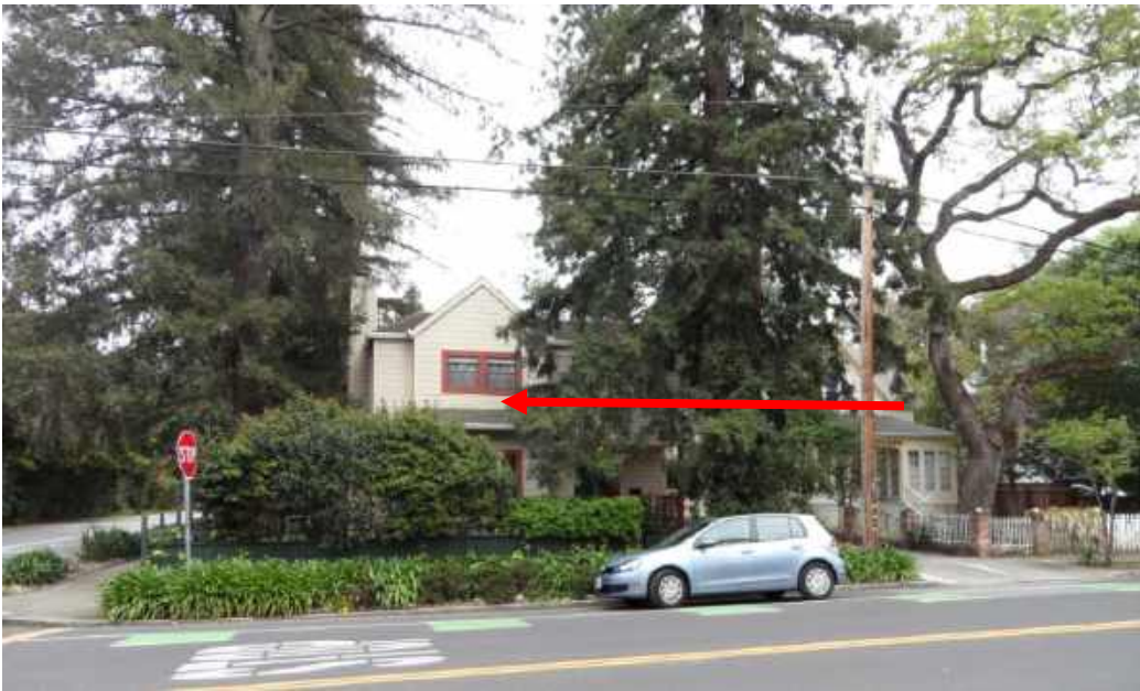
The existing building on the corner would be demolished and 417 Glenwood (on the right) would be moved to the (left) to sit on the corner.
