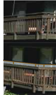
PROPOSED GUARDRAIL NEW ADDITION TO LOWER LEVEL GUARDRAIL TO BE SIMILAR AT THE SECOND STORY EXISTING GUARDRAIL
