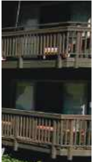
EXISTING GUARDRAIL 2ND STORY GUARDRAIL ALREADY EXTENDED
