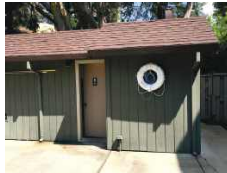
EXISTING BUILDING MEN RESTROOM
