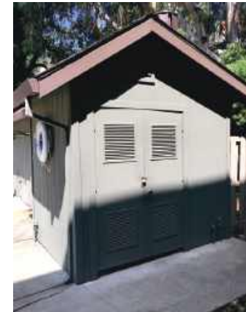
EXISTING BUILDING SIDE VIEW
