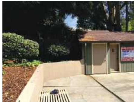
EXISTING BUILDING WOMEN RESTROOM
