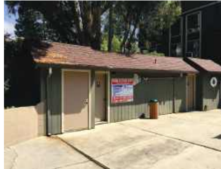
EXISTING BUILDING GENERAL VIEW (BUILDING TO BE REMOVED)
