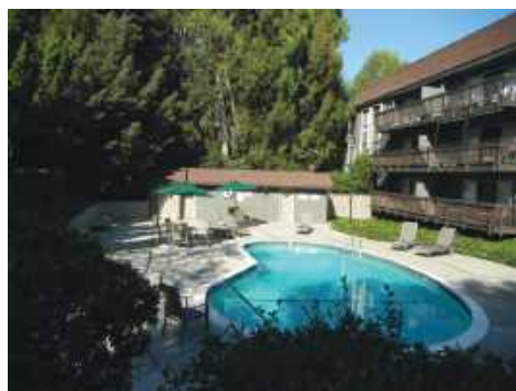
PHOTO OF EXISTING CONDITION
