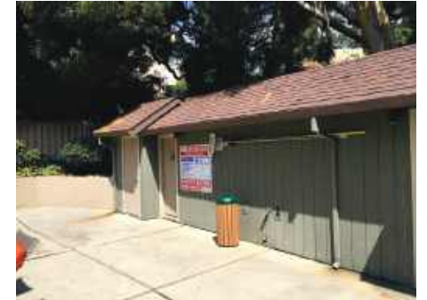
EXISTING BUILDING PARTIAL FRONT VIEW
