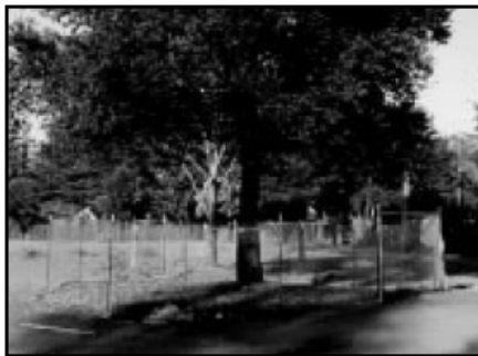
IMAGE 2.15-2 Tree Protection Fence at the Dripline
