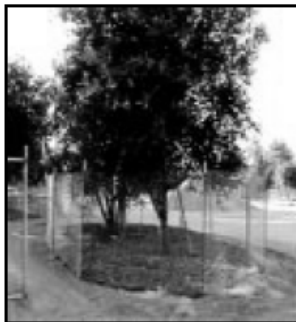
IMAGE 2.15-1 Tree Protection Fence at the Dripline
