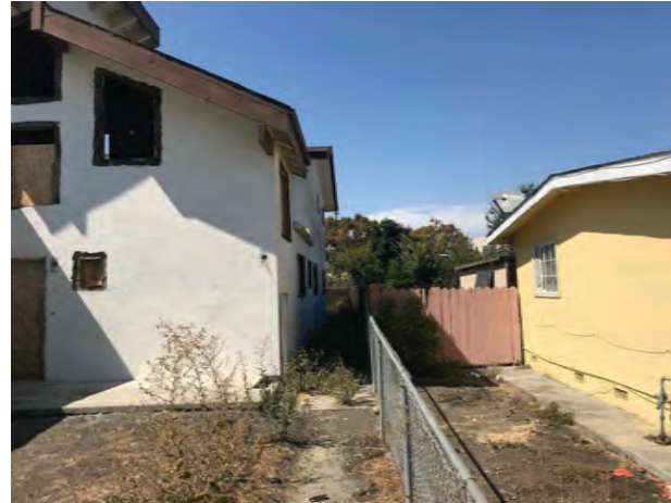
EXISTING CONDITIONS AT NORTH SIDE YARD
