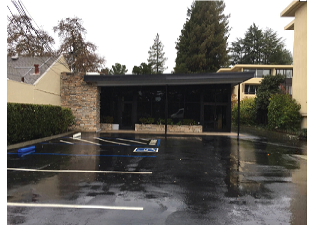
Building - Existing Condition
