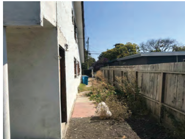
EXISTING CONDITIONS AT SOUTH SIDE YARD
