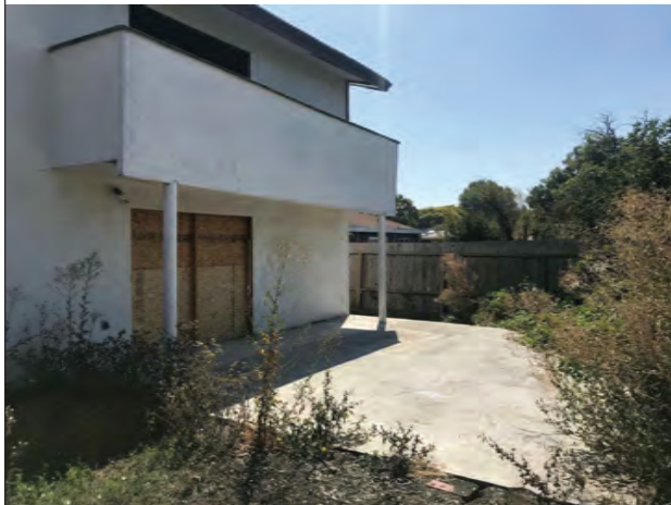
EXISTING CONDITIONS AT REAR YARD
