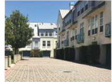
SHARED COURTYARD SPACE
