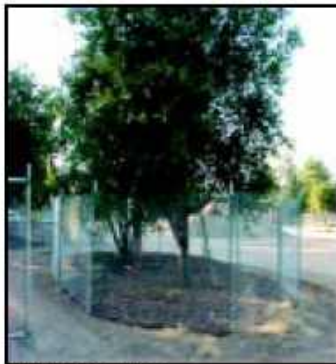
IMAGE 2.15-1 Tree Protection Fence at the Dripline
