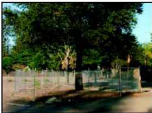
IMAGE 2.15-2 Tree Protection Fence at the Dripline
