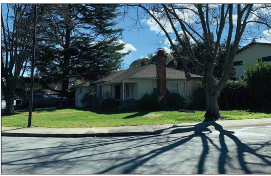
EXIST'G HOUSE NORTHWEST PHOTO
