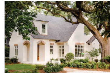
WHITE PAINTED BRICK WALLS
