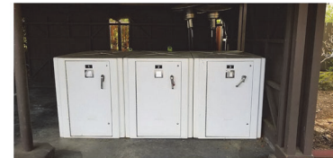
Existing bike lockers to be relocated and reuse
