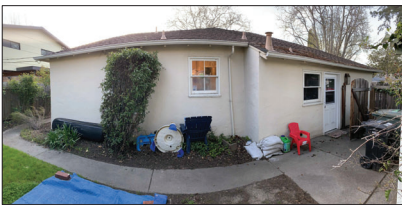
EXIST'G HOUSE SOUTHEAST (REAR) PHOTO
