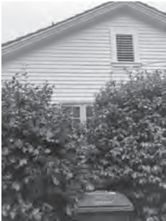
LEFT (NORTHEAST) SIDE OF HOUSE (DETAIL OF GABLE)
