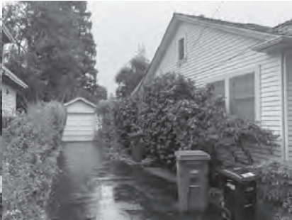
LEFT (NORTHEAST) SIDE OF HOUSE
