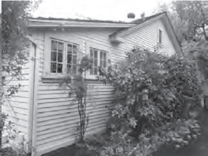
LEFT (NORTHEAST) SIDE OF HOUSE
