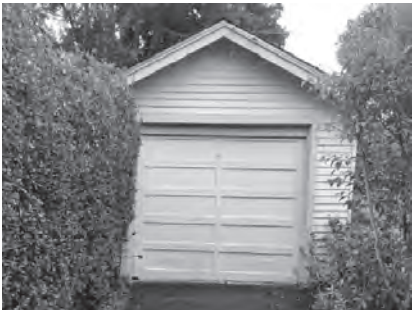
FRONT (NORTHWEST) SIDE OF GARAGE
