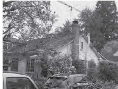
RIGHT (SOUTHWEST) SIDE OF HOUSE
