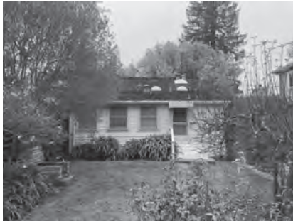
REAR (SOUTHEAST) SIDE OF HOUSE
