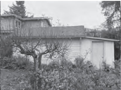
RIGHT (SOUTHWEST) SIDE OF HOUSE
