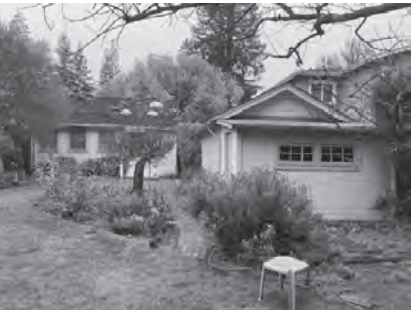
REAR (SOUTHEAST) SIDE OF GARAGE
