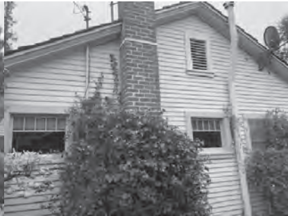
RIGHT (SOUTHWEST) SIDE OF HOUSE
