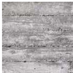
BOARD FORMED CONCRETE ③
