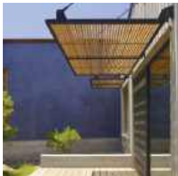
PHENOLIC WOOD AND METAL AWNING ⑧
