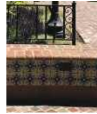
Seat Wall and Ornamental Fence
