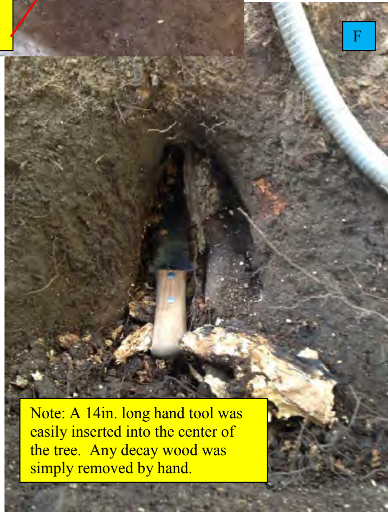
Photo F below was taken on the South side.
