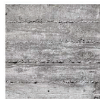
BOARD FORMED CONCRETE (3)
