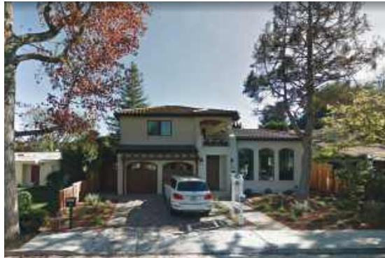
EXISTING NEIGHBORHOOD HOUSE - 715 CAMBRIDGE 5.
