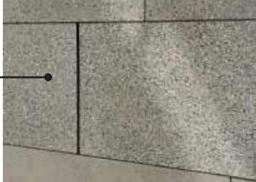
TYPE 4. CONCRETE UNIT PAVERS HEAVY SANDBLAST 24"X36"
