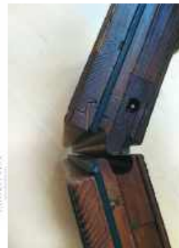
TOP VIEW OF CASEMENT COMING TOGETHER
