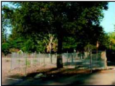
IMAGE 2.15-2 Tree Protection Fence at the Dripline
