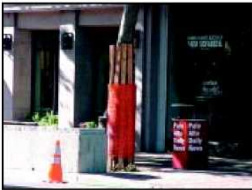
IMAGE 2.15-4 Trunk Wrap Protection
