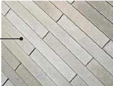
TYPE 3. CONCRETE UNIT PAVERS LIGHT SANDBLAST 3"X18"
