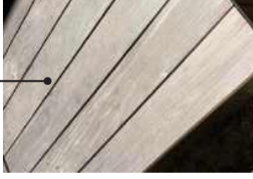
TYPE 5. WOOD DECKING THERMALLY MODIFIED WOOD
