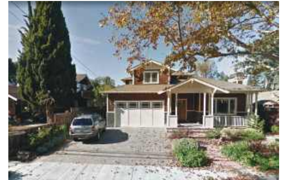
EXISTING NEIGHBORHOOD HOUSE - 680 CAMBRIDGE 3.
