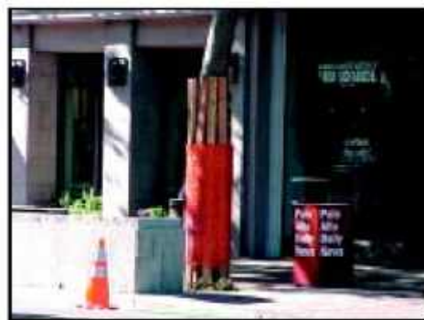
IMAGE 2.15-4 Trunk Wrap Protection
