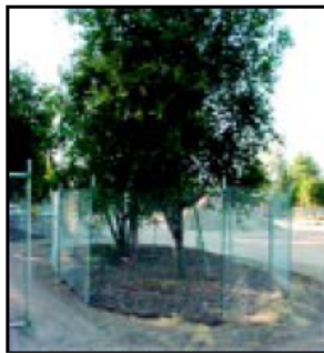
IMAGE 2.15-1 Tree Protection Fence at the Dripline
