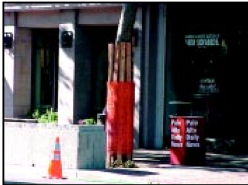
IMAGE 2.15-4 Trunk Wrap Protection
