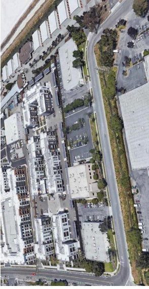
FULL LENGTH OF HAVEN AVE FRONTAGE
