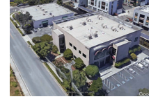
ADJACENT OFFICE BUILDING ON SOUTH
