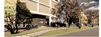
VIEW FROM PATH TO HOTEL ENTRY
