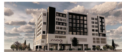
FRONT FACADE , VIEW LOOKING WEST
