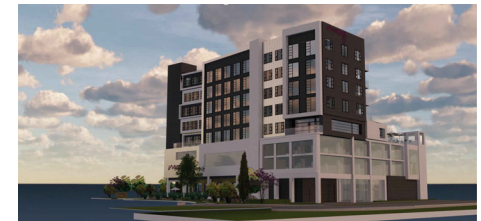
FRONT FACADE , VIEW LOOKING SOUTHWEST
