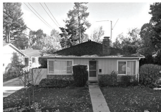
2 N.T.S. PHOTO OF EXISTING FRONT FACADE
