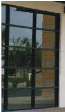
storefront system dark metal lobby
