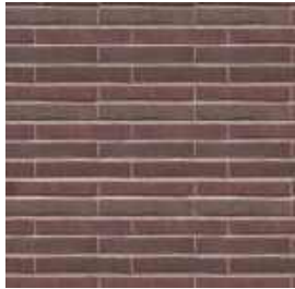
glazed brick (fireclay tile or similar) street level walls
