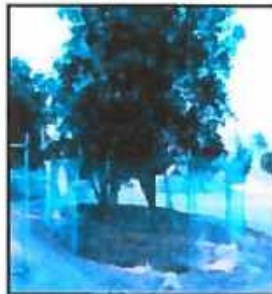
IMAGE 2.15-1 Tree Protection Fence at the Dripline
