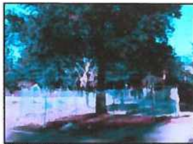
IMAGE 2.15-2 Tree Protection Fence at the Dripline
