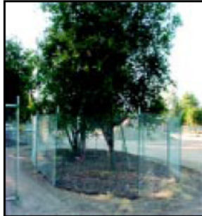
IMAGE 2.15-1 Tree Protection Fence at the Dripline
