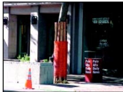
IMAGE 2.15-4 Trunk Wrap Protection
