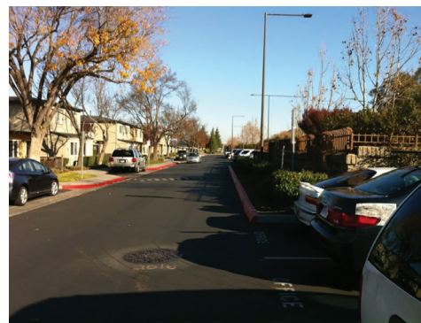
6. LOOKING NORTH ALONG FRONTAGE RD.
