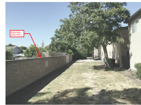
7. TYPICAL REAR YARD VIEW
