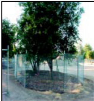
IMAGE 2.15-1 Tree Protection Fence at the Dripline
